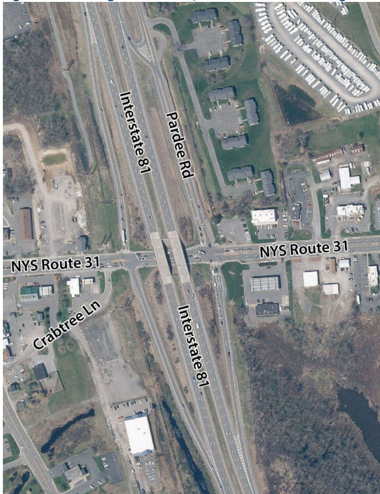
Figure 5-2: Existing Interstate 81/NYS Route 31 Interchange
