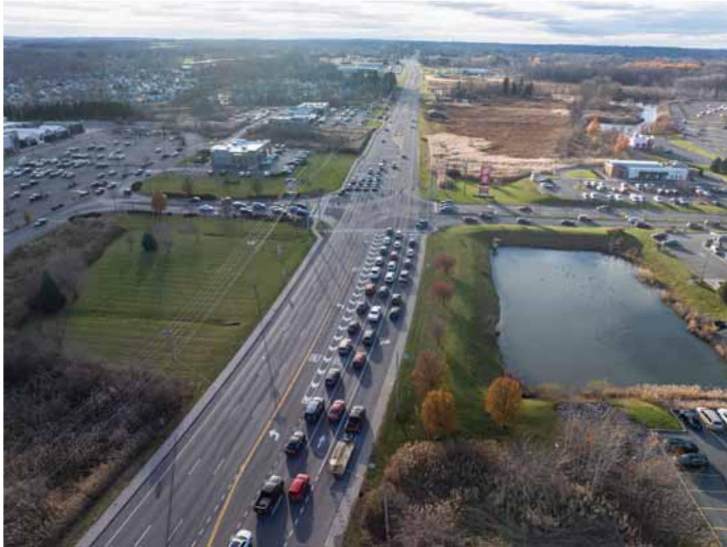
NYS Route 31 at Dell Center Drive Intersection November 2025
