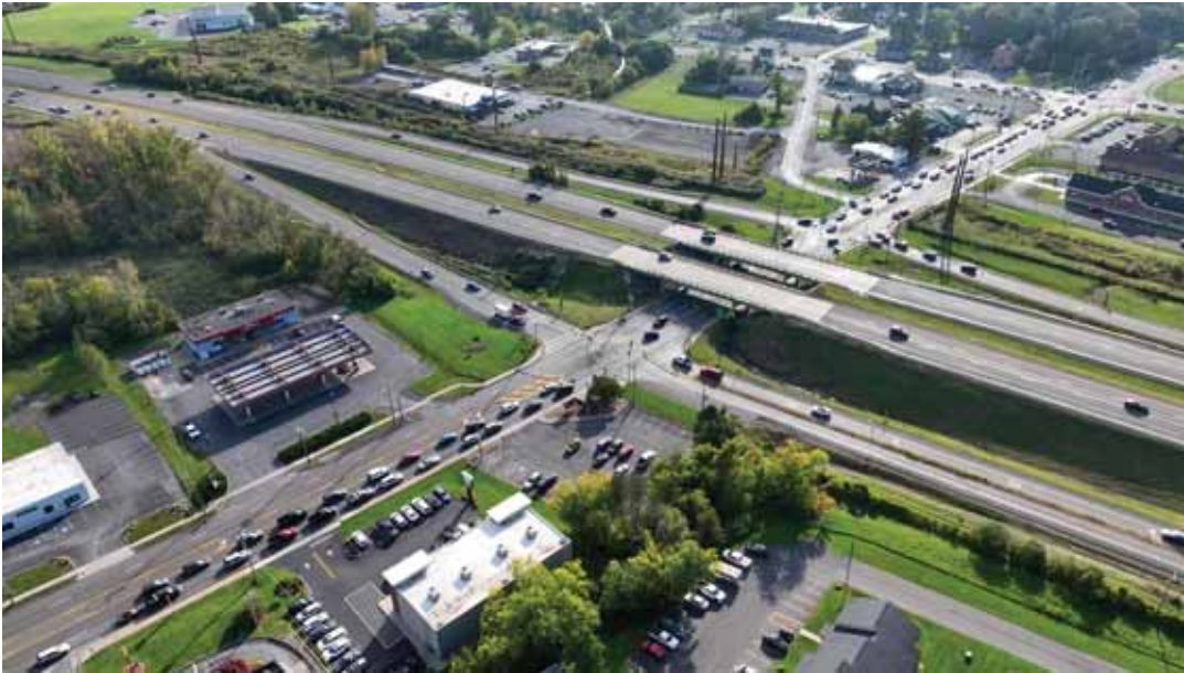
NYS Route 31 at Interstate 81 Interchange
