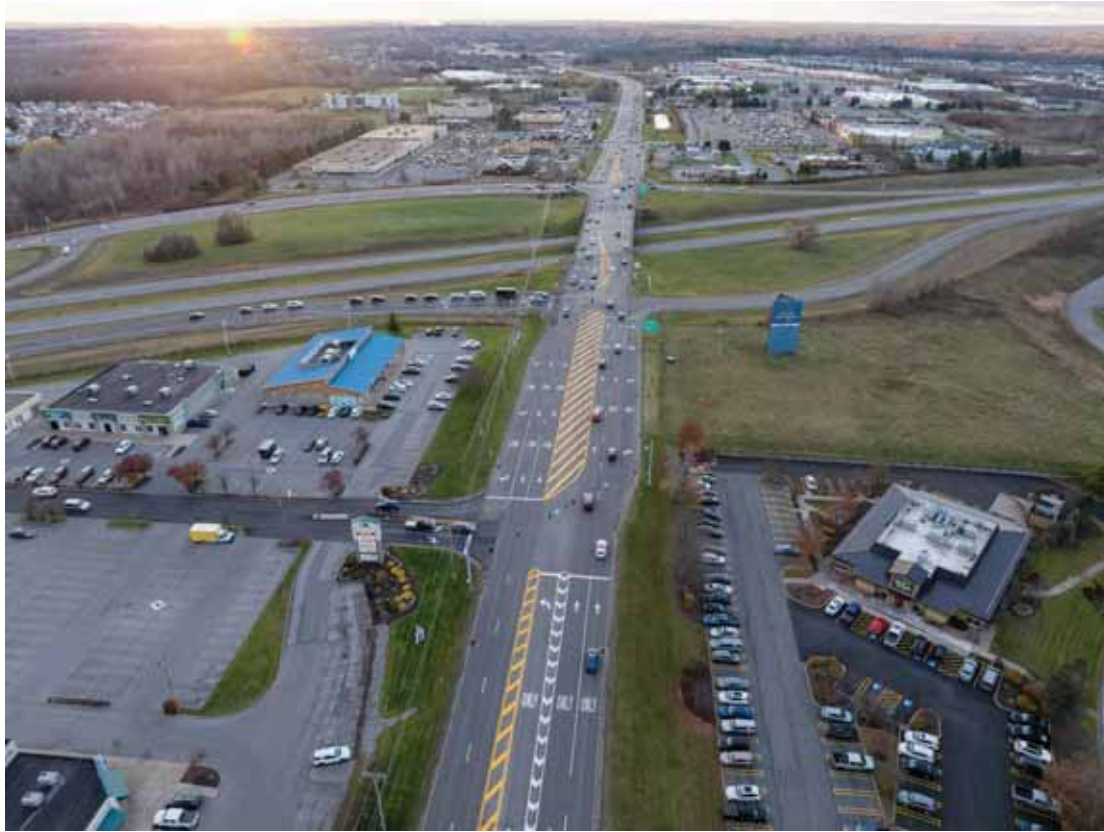
NYS Route 31 at NYS Route 481 Interchange November 2025
